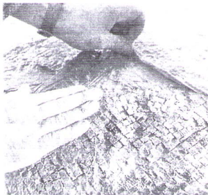
Mr. Piras peeling away a glued paper holding pieces of tile, setting them in the section of concrete.
